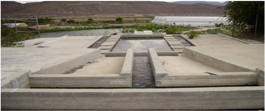
Figura 15. Tanque imhoff.
