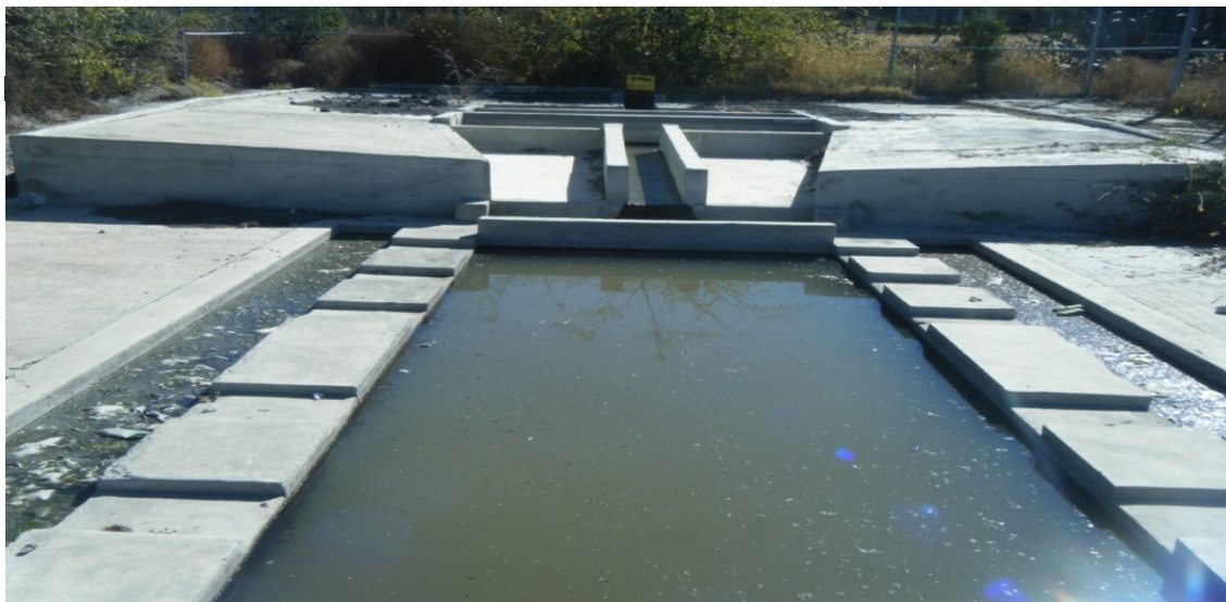
Figura 7. Tanque Imhoff.
