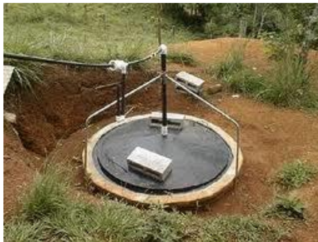
FIGURA 2. DIGESTOR SEMI- CONTINUO
