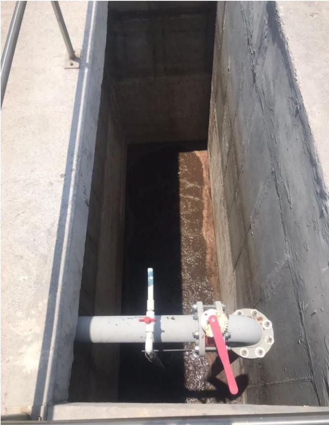
Figura 2. Digestor Aerobio (PTAR-UAAAN, 2022).
