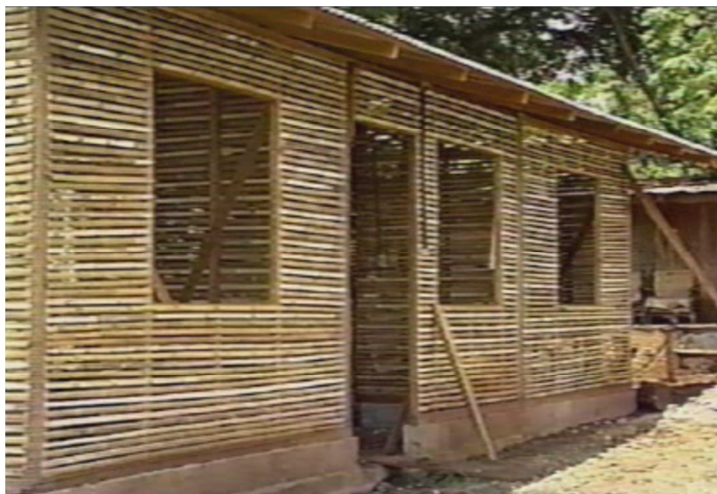
©FUMBAMBU, paneles sin rellenar, 1995
