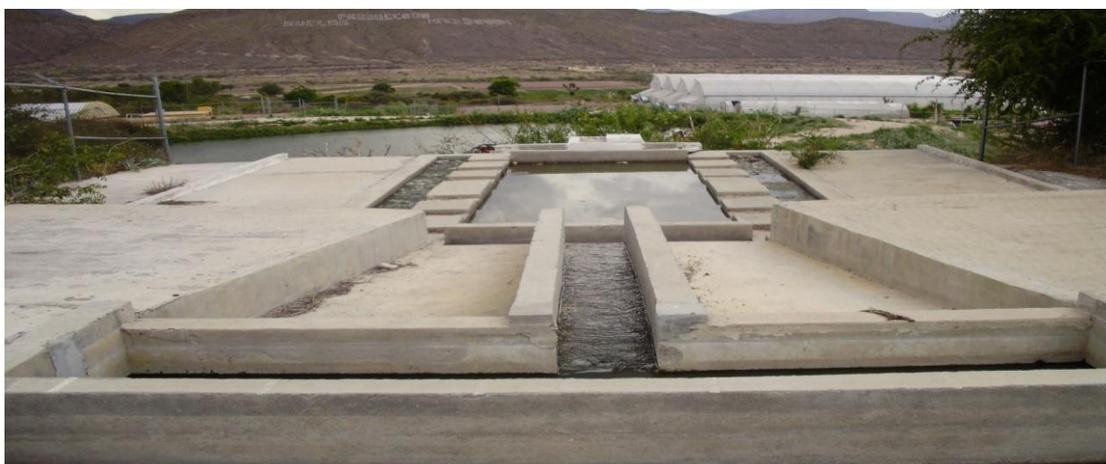
Figura 12. Tanque Imhoff
