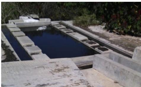
Figura 3.6. Tanque Imhoff.
